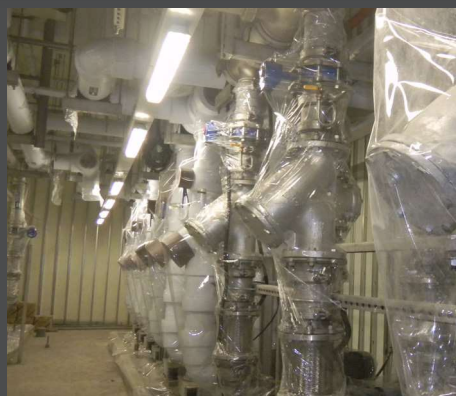
KEELUNG RAILWAY STATION Keelung City, Taiwan
