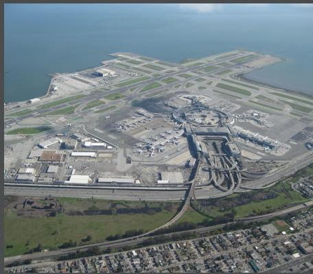
SAN FRANCISCO INT. AIRPORT San Francisco, California
