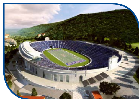
California Memorial Stadium Berkeley, CA
