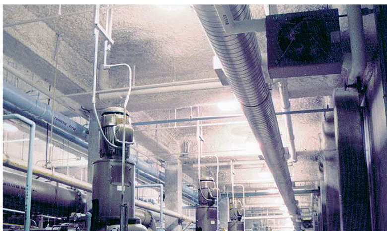
NEW BEDFORD WASTE WATER TREATMENT PLANT - NEW BEDFORD, MA, USA | K-13 White | 30,000 sf - 3" Thick
